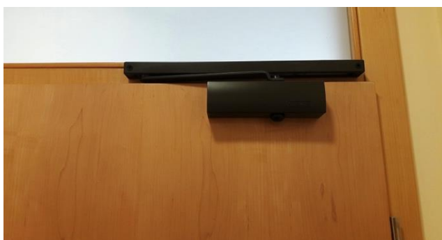
Slika 14: door self-closing mechanism
