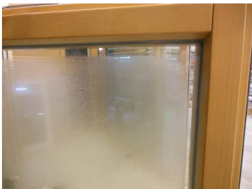
Slika 58: Steaming up of external glass
