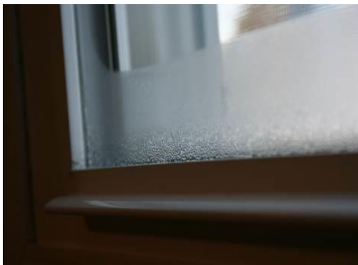
Slika 57: Steaming up of internal glass
