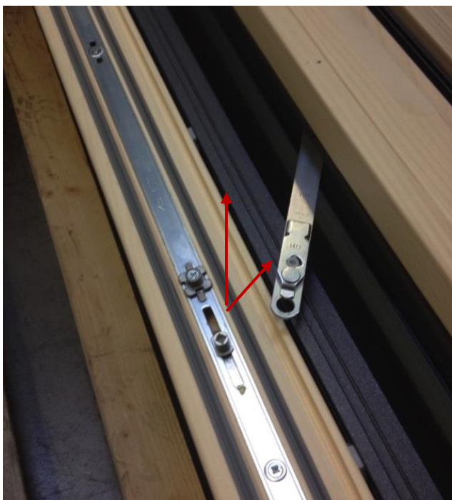
Slika 45: Releasing the scissors by pulling up
