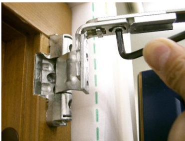
Slika 24: Tightening of the upper part of the window (top hinge)
