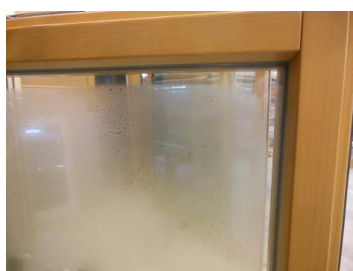
Image 62: Steaming up of external glass
