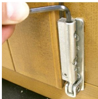
Slika 20: Height adjustment of window (bottom hinge)
