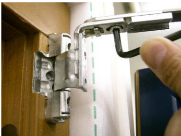
Slika 24: Tightening of the upper part of the window (top hinge)
