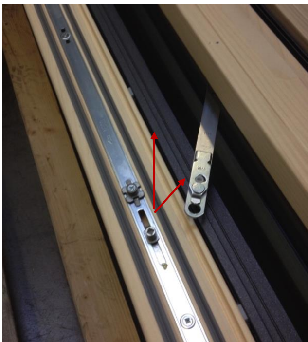
Slika 45: Releasing the scissors by pulling up
