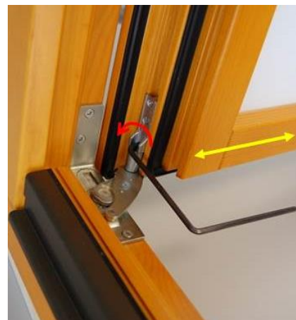
Slika 32: Horizontal movement (bottom)
