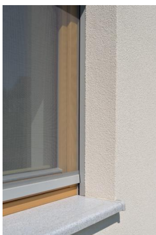
Slika 16: retractable insect screen
