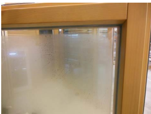
Slika 58: Steaming up of external glass
