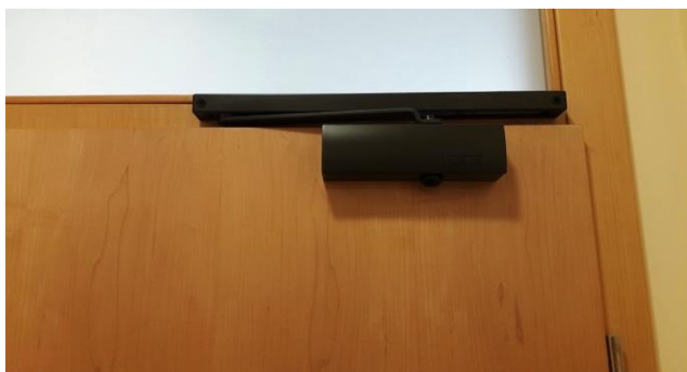
Slika 14: door self-closing mechanism
