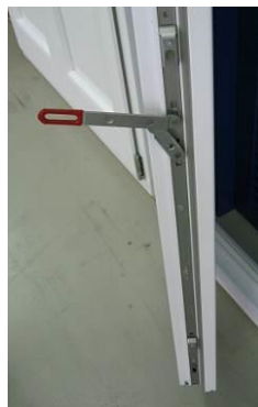
Slika 3: Mechanism for opening double-sash window or balcony door without a mullion
