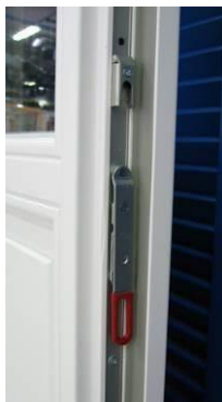
Slika 3: Mechanism for opening double-sash window or balcony door without a mullion
