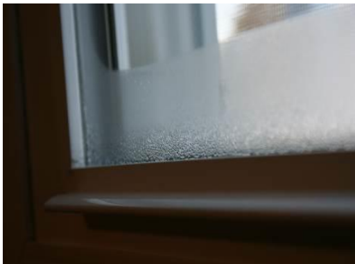
Slika 57: Steaming up of internal glass
