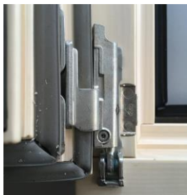
Slika 21: Moving the sash to the frame (bottom hinge)
