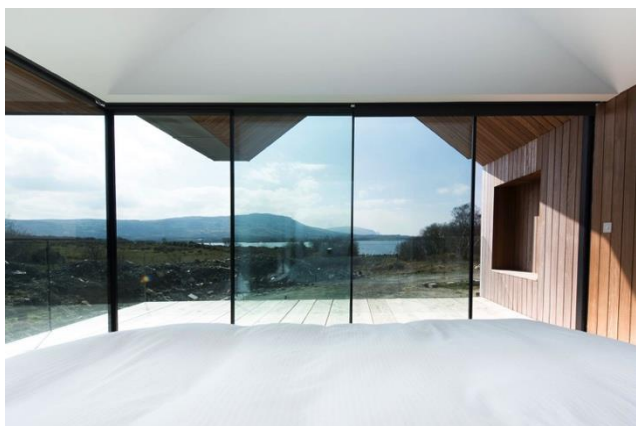
Slika 8: Glass corners and large fixed glazing
